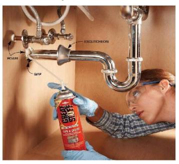
Pull back the escutcheons on plumbing pipes where they enter exterior walls and you'll probably see generous gaps around the pipes. In cold weather, you might also feel the draft coming in. All it takes is a can of expanding foam to seal those leaks.
